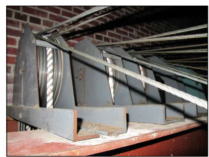
EXISTING HEAD BLOCKS
