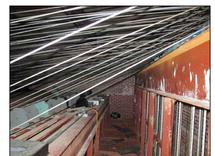
EXISTING LOFT BLOCKS & LOADING BRIDGE
